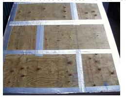
Figure A-3. Self-Adhering Modified Bitumen Strips Applied to Plywood Joints of Roof Deck
