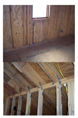
Figure 2-41. Framing and Connection Details for FBC Gable Roof Home.
