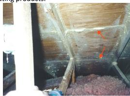
Figure A-4. Sprayed on Structural Adhesives to Seal Plywood Joints (SWR) and Strengthen Roof Deck Attachment
