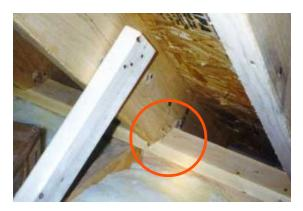
Figure A-5. Example of a Toe-Nail Connection Used for Rafter-to-Top Plate Connection
