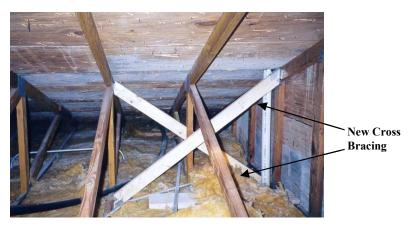
Figure A-10. Gable End Bracing Secured with Metal Connections.
